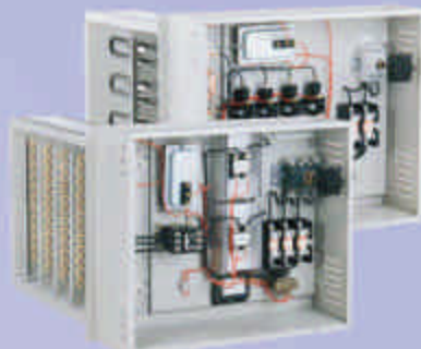
Repair or Rebuilding of Electrical Duct Heaters
